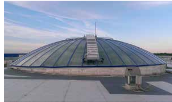
One of the semicircular head ends of the street light with the glass of the new bridge maintenance.
